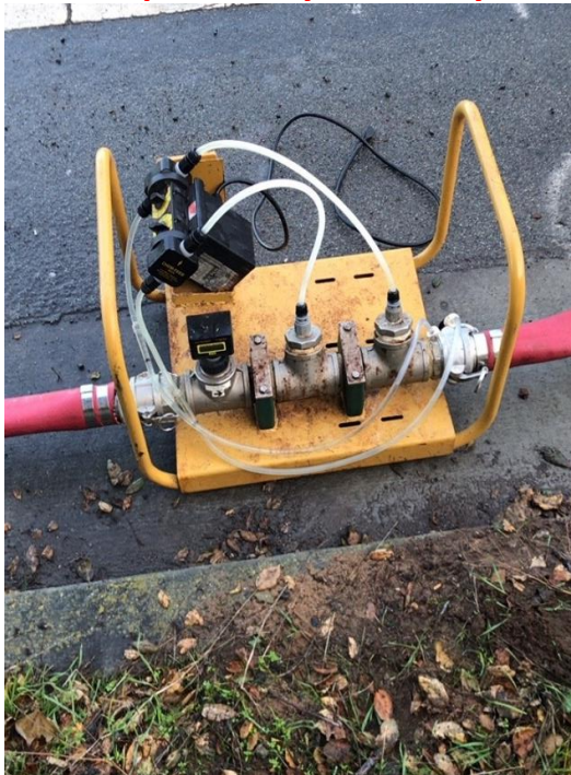
Chlorine injection for disinfection
